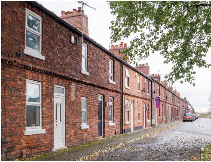
← Tilford Road, Newstead. Terraces built by the Newstead Colliery Company for miners, sometime between 1875 and 1885.
