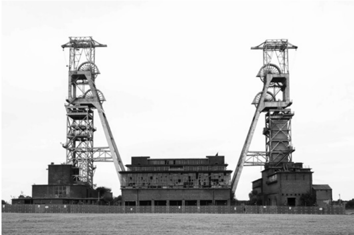
† Clipstone Colliery headstocks, the most impressive site in the Nottinghamshire coalfield and Grade II listed in 2000.
